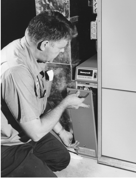
Fig. 29. Close access door to complete air cleaner installation.
