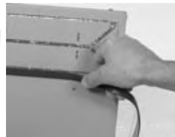
figure 2.2h - Apply plenum seal tape all around both openings on the back of the unit.
