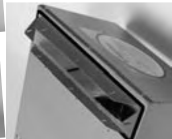
figure 2.2j- Bend tabs outward approximately 90 degrees.
