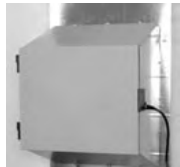
figure 2.4b - Replace door and insert power cord into the receptacle of the filter units and the other end into wall outlet.
