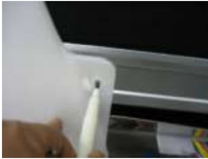
Mark the location to drill the hole. Make sure the bottom of the vent will align with the bottom of the front door panel.
