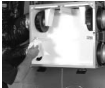
figure 17.4 Wash the Walls of the Unit
