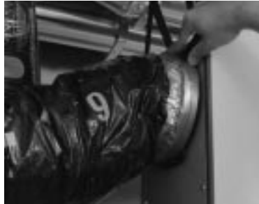
figure 7.5 Slide collar on the unit.
