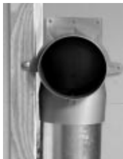
figure 11.2 Stack head elbow.
