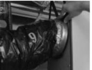
figure 7.5 Slide collar on the unit.
