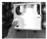
figure 17.4 Wash the Walls of the Unit
