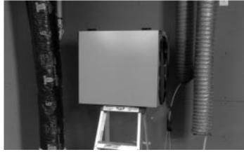
figure 5.1 Place HRV/ERV on a stepladder.
