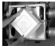
figure 17.3 Slide out the Energy Core
