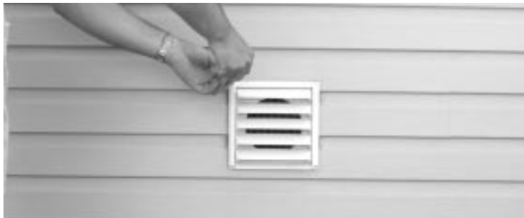
figure 10.4 Install outside hoods.
