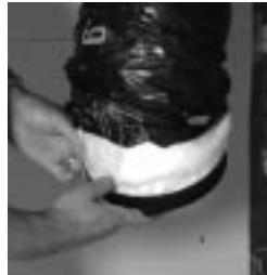
figure 7.3 Insert insulation inside the collar.
