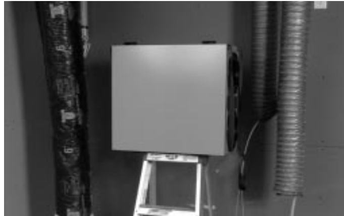
figure 5.1 Place HRV/ERV on a stepladder.
