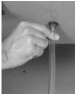
figure 8.2 Insert condensate line.
