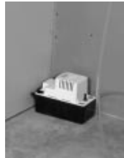
figure 8.4 Use a condensate pump if you don't have access to the floor drain.
