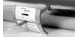
figure 13.4 Inserting Air flow grid in duct
