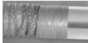
figure 6.2 Mount flex to rigid duct.
