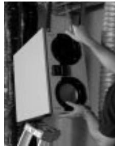
figure 5.3 Pull on the middle strap and gently push upward on the unit. Then repeat procedure on other side.
