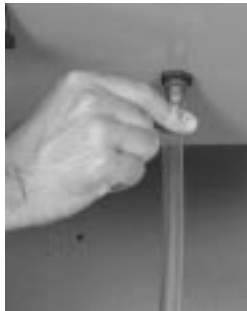
figure 8.2 Insert condensate line.
