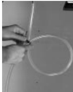
figure 8.3 Make a loop in condensate line.
