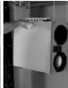
figure 5.4 When completing the procedure make sure that the HRV or ERV is leveled.
