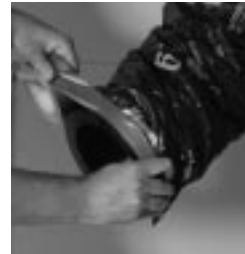
figure 7.4 Finish by taping the duct on the collar.
