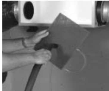
figure 17.2 Vacuum the Filters
