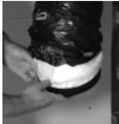
figure 7.3 Insert insulation inside the collar.
