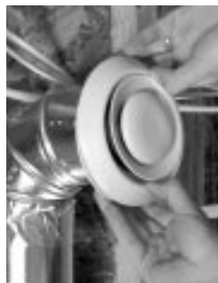
figure 11.3 Insert grille.
