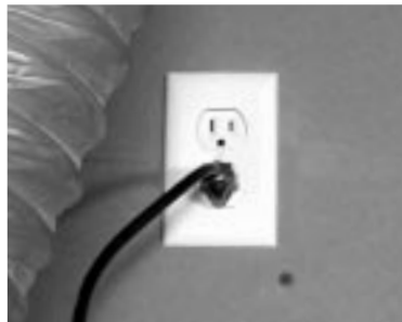
figure 9.2 Electric Wall Outlet
