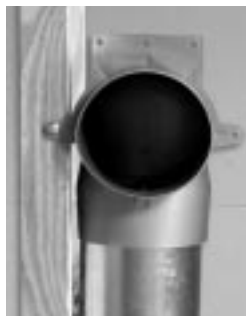
figure 11.2 Stack head elbow.
