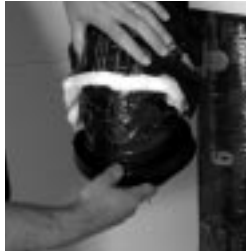
figure 10.2 Insert vinyl duct over the hooks. Fix the collar on the floor joist.
