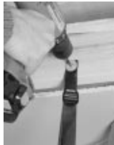
figure 5.2 Attach your four straps to the floor joist making sure that you attach thru the washers and the grommets.
