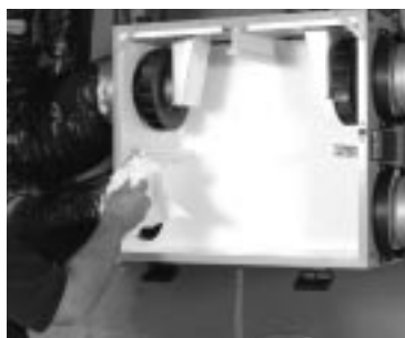
figure 17.4 Wash the Walls of the Unit
