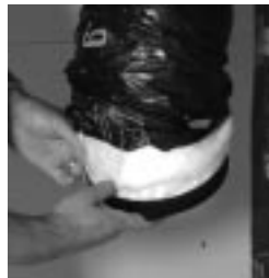
figure 7.3 Insert insulation inside the collar.
