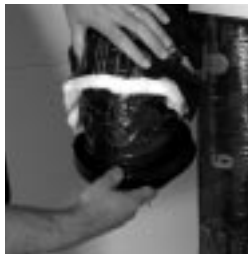
figure 7.2 Insert vinyl duct over the hooks and seal with a 30" tie wrap.
