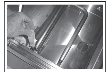
Install burner. Tighten screw.
