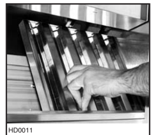
BAFFLE FILTER (TYPICAL)
