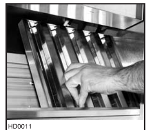
BAFFLE FILTER (TYPICAL)
