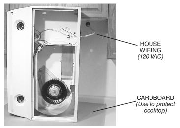
Connect <u>House Wiring</u> (120 VAC) to hood. Use a piece of <u>Cardboard</u> to protect the cooktop, if necessary.
