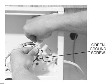
Connect house black to hood black wire, house white to hood white wire, and house ground under **Green Ground Screw**. Securely tighten cable clamp onto house wiring.
