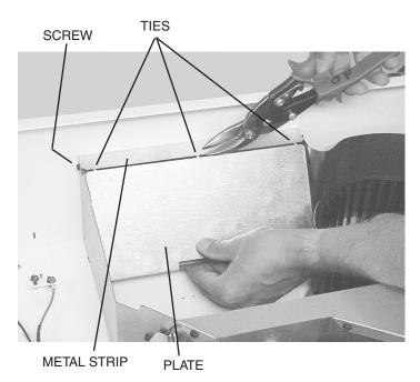
Horizontal Discharge Only: Remove the <u>Plate</u> in front of the horizontal discharge knockout. Cut the <u>Ties</u>, lift plate out, and discard plate. DO NOT REMOVE the <u>Metal Strip</u> held in place with two **Screws**.
