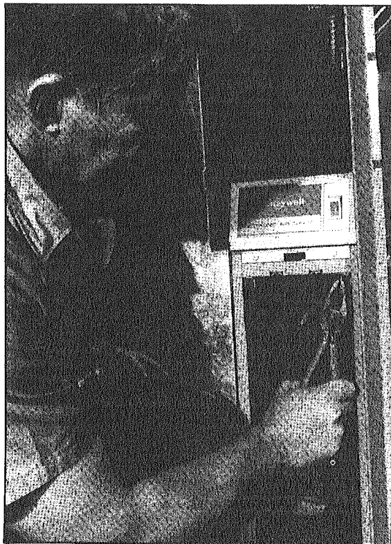
FIG. 17—CRIMP END OF UNUSED CHANNELS.
