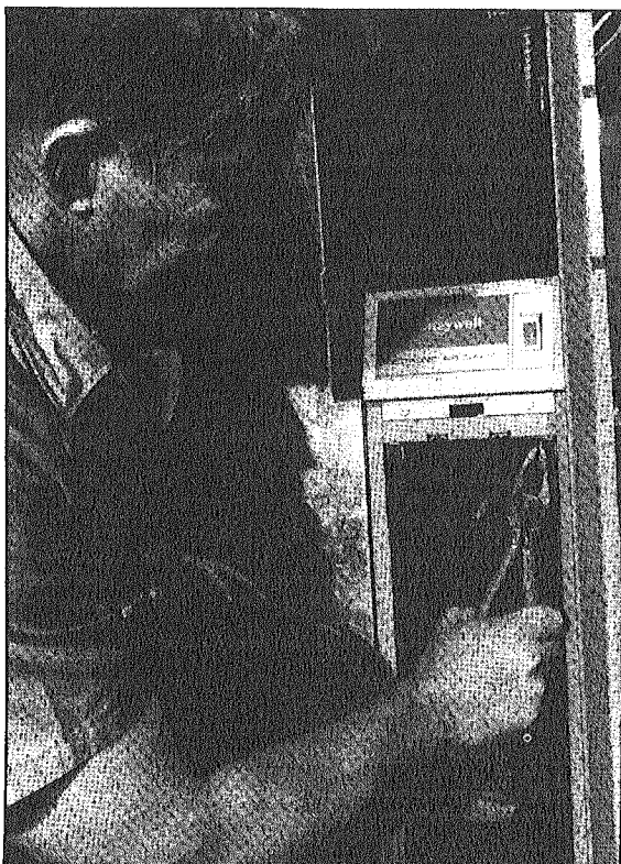
FIG. 17—CRIMP END OF UNUSED CHANNELS.
