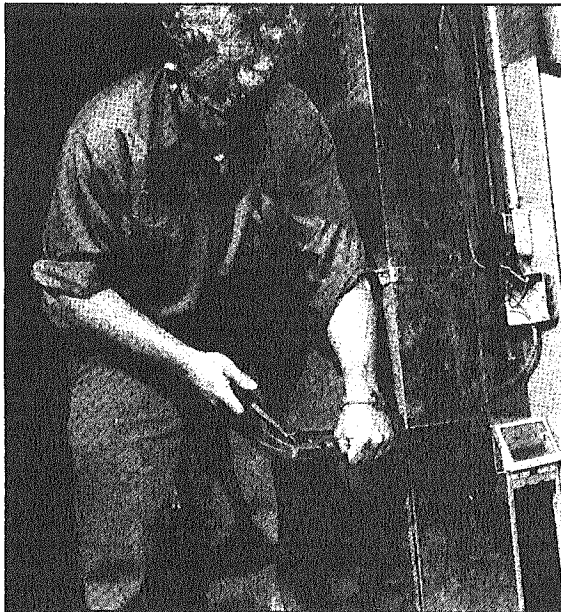
FIG. 16—COMPLETE THE DUCT INSTALLATION.
