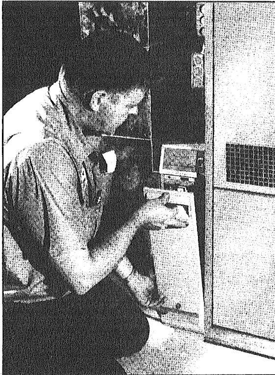
FIG. 22—ACCESS DOOR ACTUATES SHORTING INTERLOCK WHEN CLOSED.
