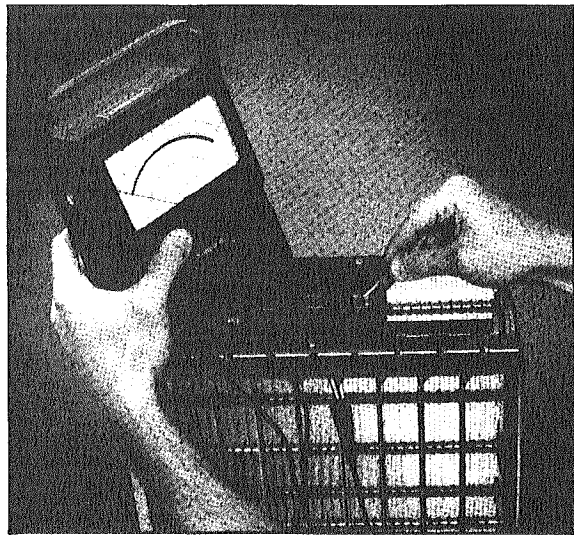
FIG. 34—USE AN OHMMETER TO CHECK THE ELECTRONIC CELLS FOR SHORT CIRCUITS.
