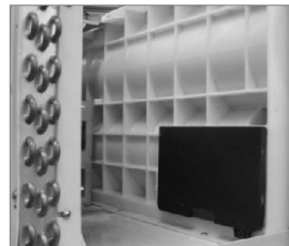
Figure B – Vent Filter Removal
