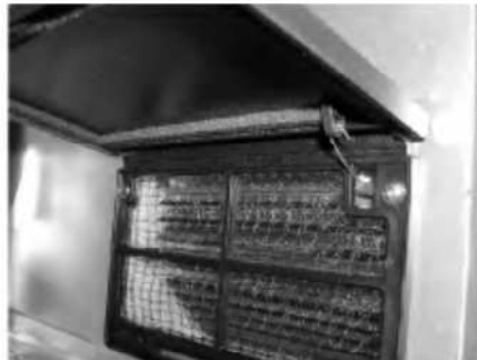
Figure 16 – Vent Filter Removal
