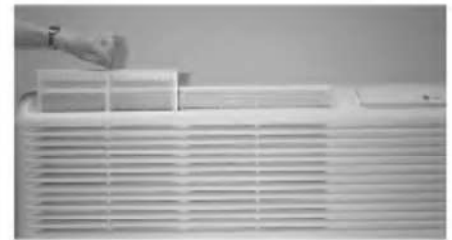
Figure 14 - Filter Removal
