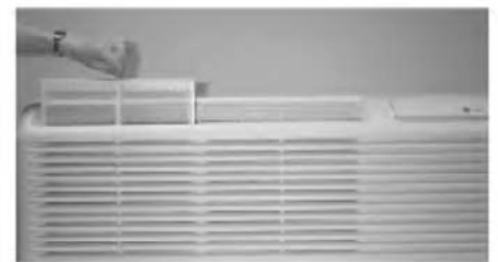
Figure 14 - Filter Removal
