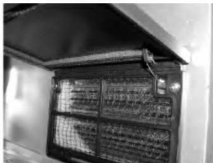
Figure 16 – Vent Filter Removal
