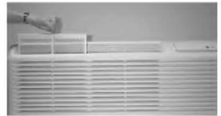
Figure 14 - Filter Removal
