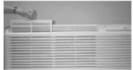
Figure 14 - Filter Removal
