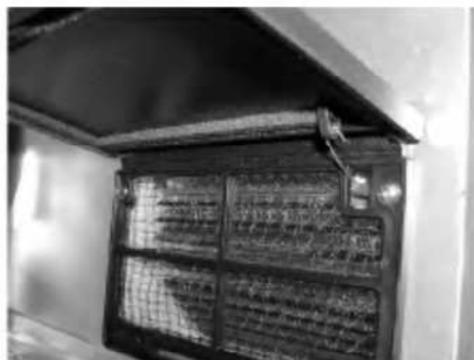
Figure 16 – Vent Filter Removal
