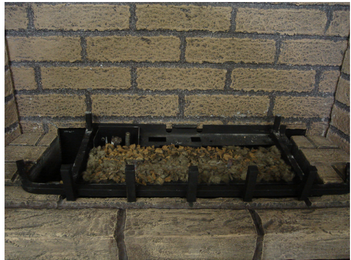
Figure 50 - Rock wool placement
