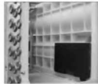
Figure B – Vent Filter Removal
