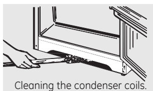
Cleaning the condenser coils.
