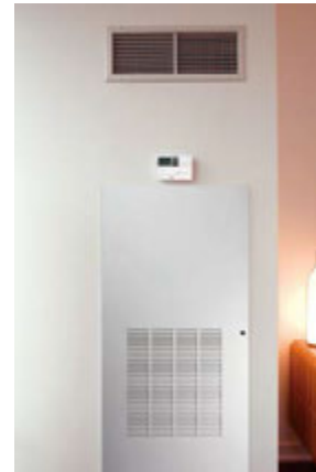
Installs in a small mechanical closet and can be ducted to multiple rooms.
