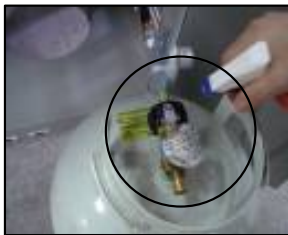
Gas Connection Leak Check
