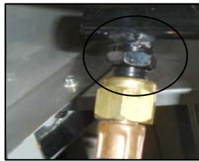
Gas Connection Leak Check
