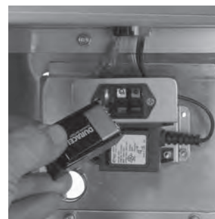
4. Insert and/or replace a new 9V battery
