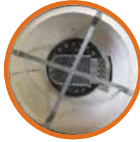
Bracket Installed Interior Fire Bowl
