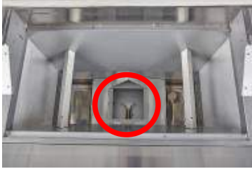
Picture 1 – Heating Element
