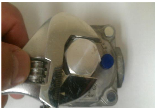
1. Remove Threaded Cap
