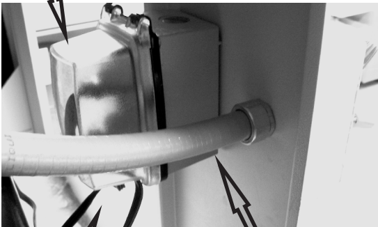
VISTA INTERIOR - PANEL CENTRAL
