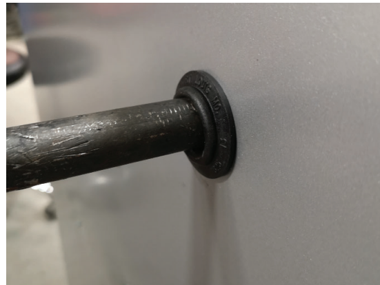
FIGURE 27 - FURNACE GAS PIPE CONNECTIONS (NOTE RUBBER GROMMET)
