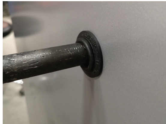
FIGURE 27 - FURNACE GAS PIPE CONNECTIONS (NOTE RUBBER GROMMET)
