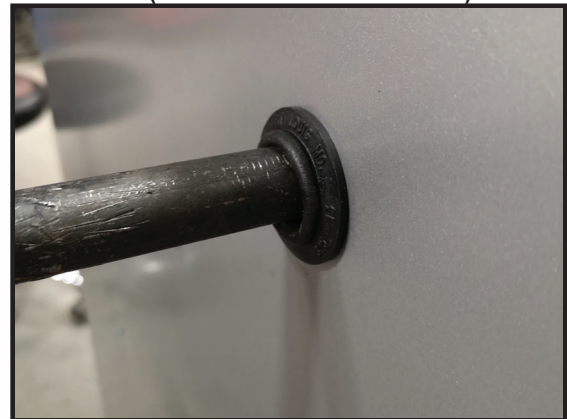
FIGURE 28 - FURNACE GAS PIPE CONNECTIONS (NOTE RUBBER GROMMET)
