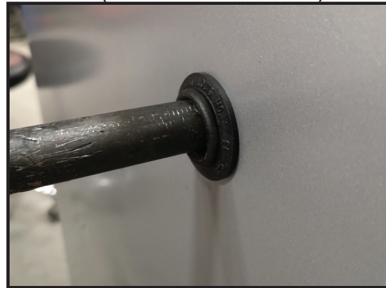
FIGURE 28 - FURNACE GAS PIPE CONNECTIONS (NOTE RUBBER GROMMET)
