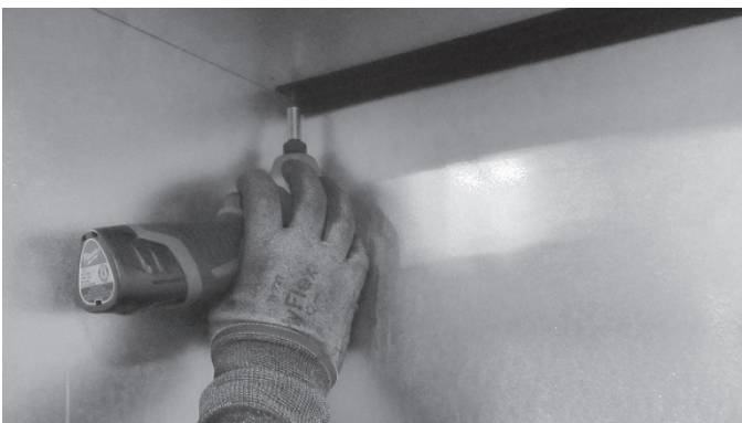
Figure 7.2 - Remove Rear Black Magic Glass Bracket
