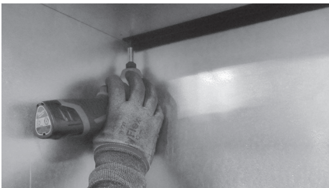
Figure 7.2 - Remove Rear Black Magic Glass Bracket
