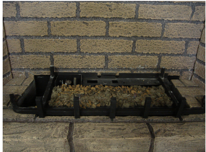
Figure 54 - Rock wool placement
