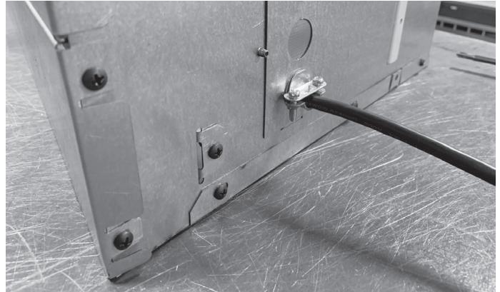
Figure 5.2 Reattaching Junction Box Cover
