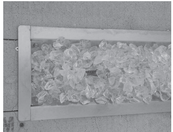
Figure 5.3 Pan Installed on Top of Finish Material
