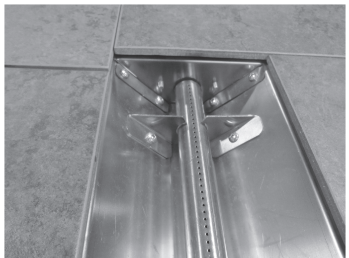
Figure 5.4 Pan Installed Under Finish Material
