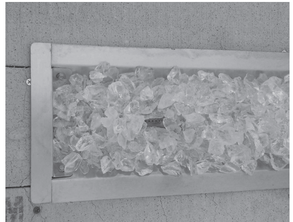
Figure 5.3 Pan Installed on Top of Finish Material
