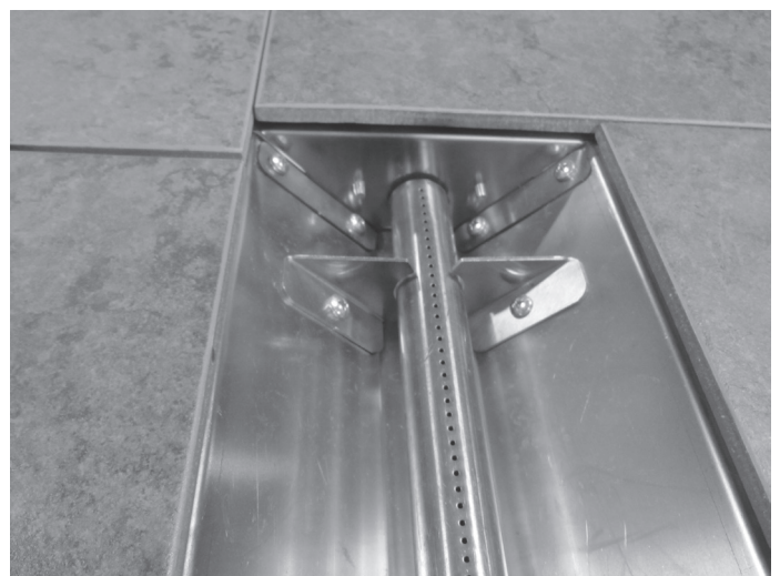
Figure 5.4 Pan Installed Under Finish Material
