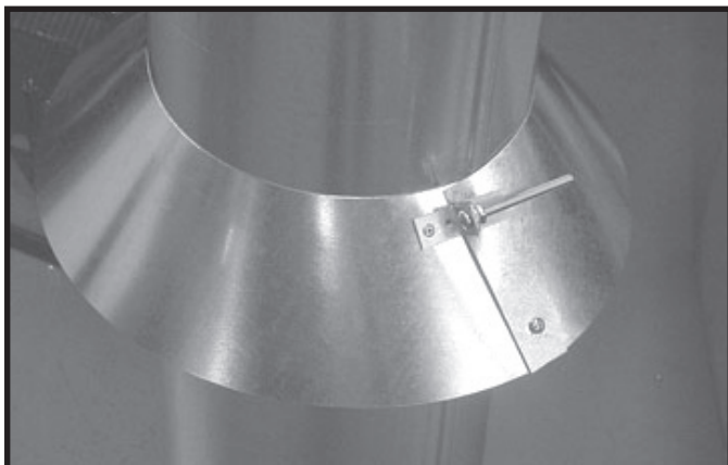
Figure 7.13 insert Bolt into Brackets
