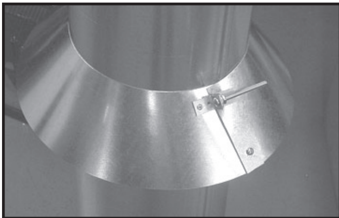
Figure 7.13 insert Bolt into Brackets
