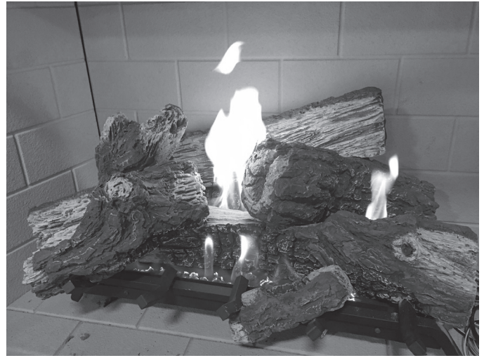
Figure 6.13 - Correct Appearance of Rear Flames
