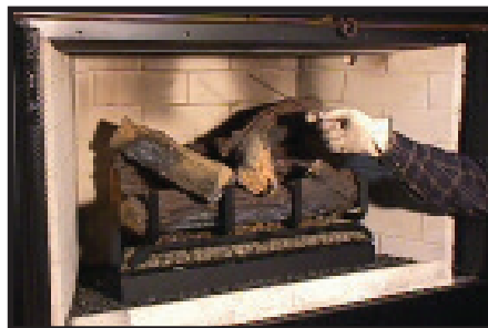
Figure 16 - Checking for Spillage
