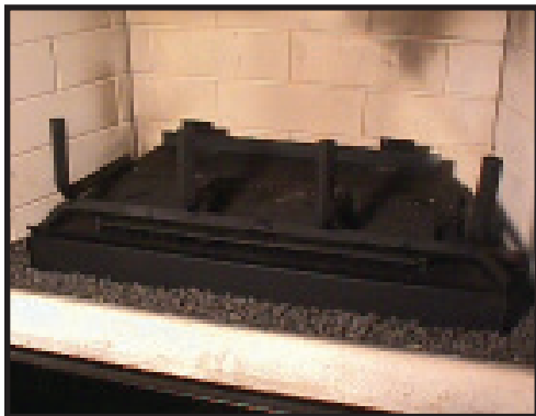
Figure 6 - Placing the Grate Assembly
