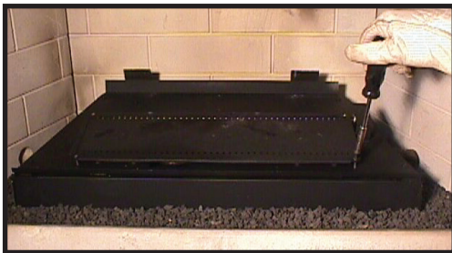
Figure 3 - Burner Assembly
