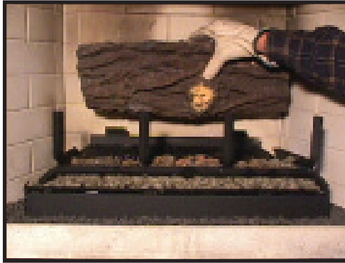
Figure 9 - Rear Log Placement
