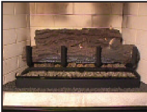
Figure 10 - Placing the Front Log
