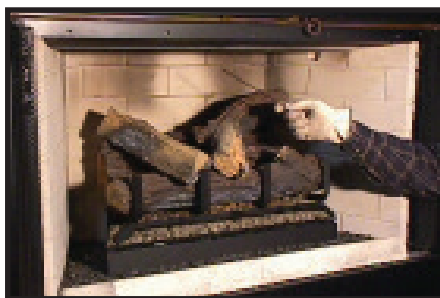
Figure 16 - Checking for Spillage
