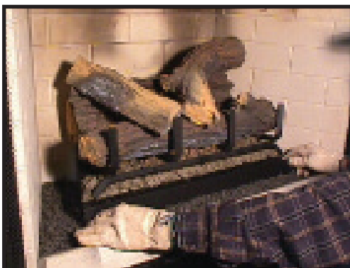
Figure 14 - Access Cover Removal
