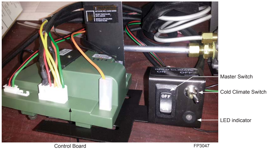
Figure 2 – 36CFDV Fireplace Controls–IPI (featuring Cold Climate option)
