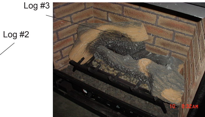
Figure 49 - Placement of Log 3
