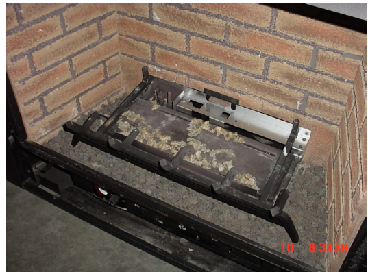
Figure 46 - Placement of Rock Wool on Burner
