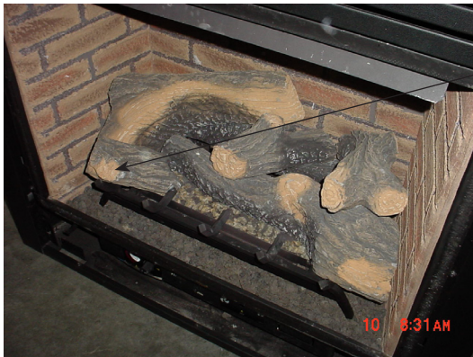
Figure 52 - Placement of Log 6
