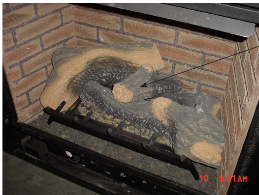
Figure 50 - Placement of Log 4
