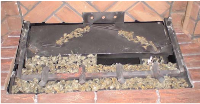
Burner Grate Assembly
