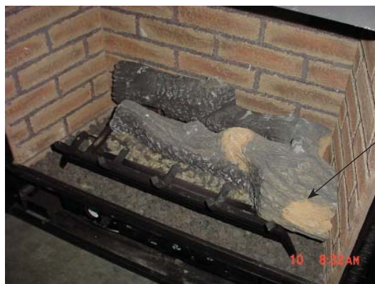
Figure 48 - Placement of Log 2
