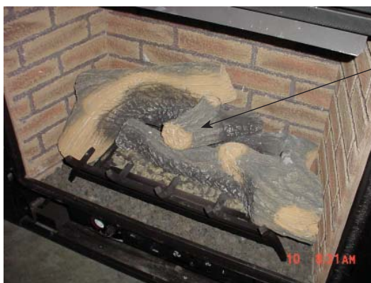
Figure 50 - Placement of Log 4
