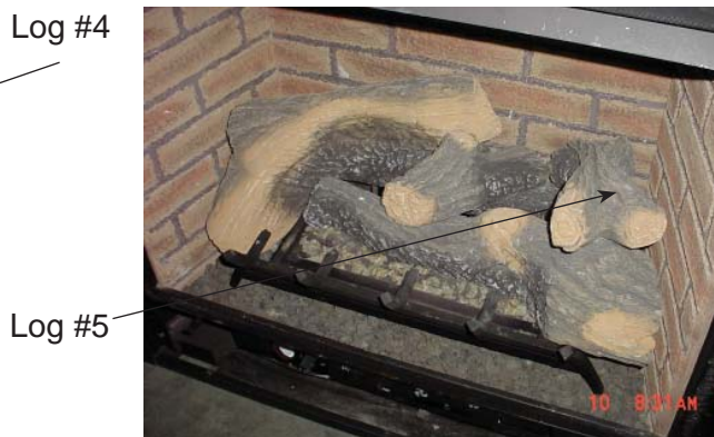
Figure 51 - Placement of Log 5
