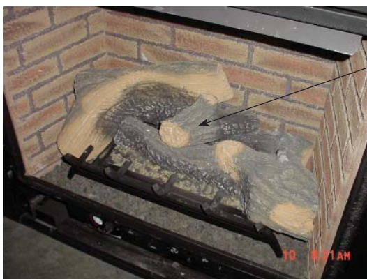
Figure 50 - Placement of Log 4
