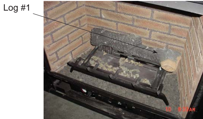
Figure 47 - Placement of Log 1.
