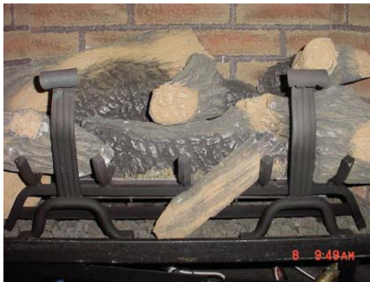
Figure 54 a & b - Andiron Placement (400DVBH and 300DVBH).
