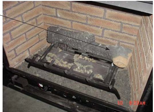
Figure 47 - Placement of Log 1.
