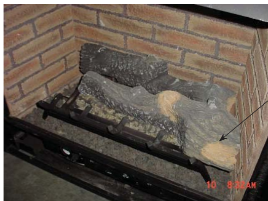
Figure 48 - Placement of Log 2
