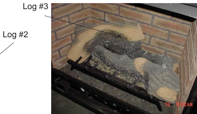
Figure 49 - Placement of Log 3
