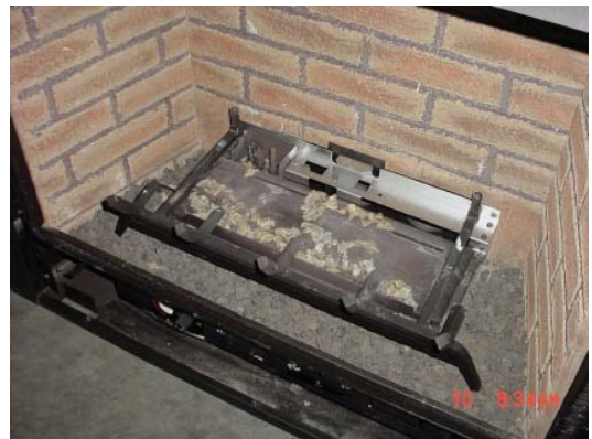
Figure 46 - Placement of Rock Wool on Burner
