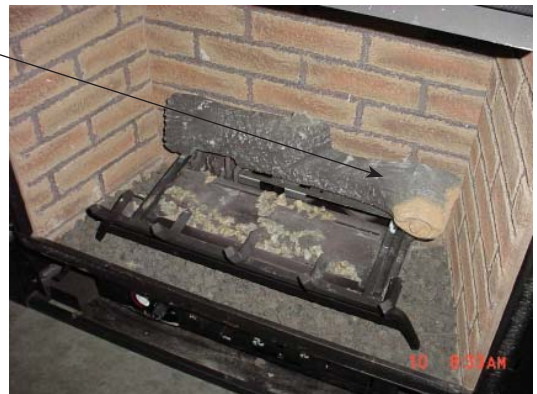
Figure 47 - Placement of Log 1.
