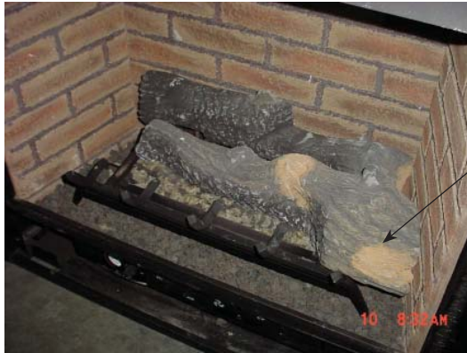
Figure 48 - Placement of Log 2
