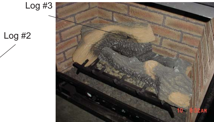
Figure 49 - Placement of Log 3
