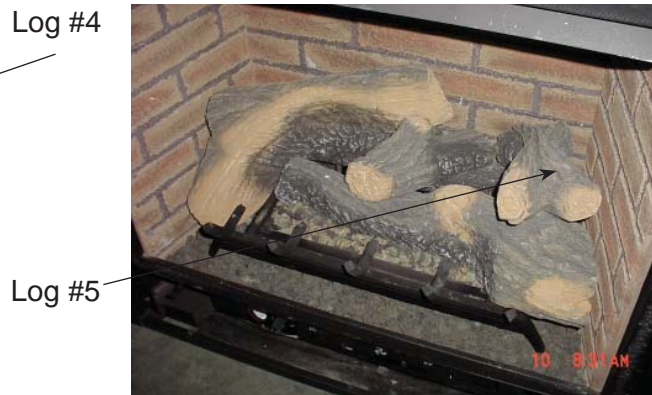
Figure 51 - Placement of Log 5
