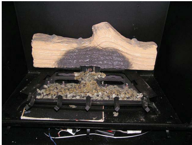
Figure 46 - Installing Rear Log
