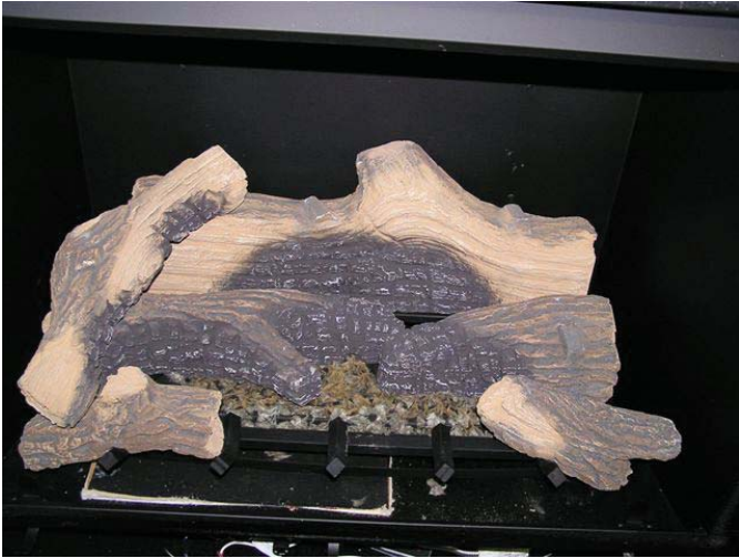
Figure 51 - Installing upper left log
