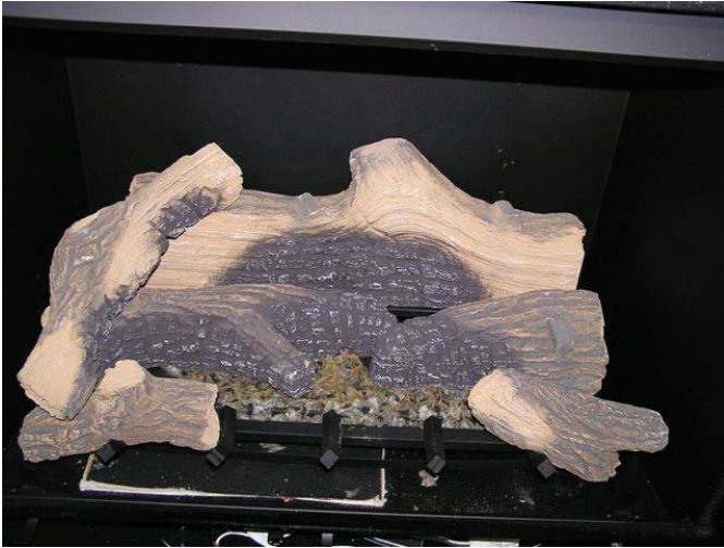
Figure 51 - Installing upper left log
