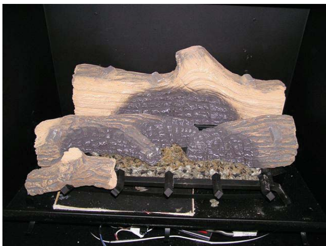
Figure 49 - Installing left front log
