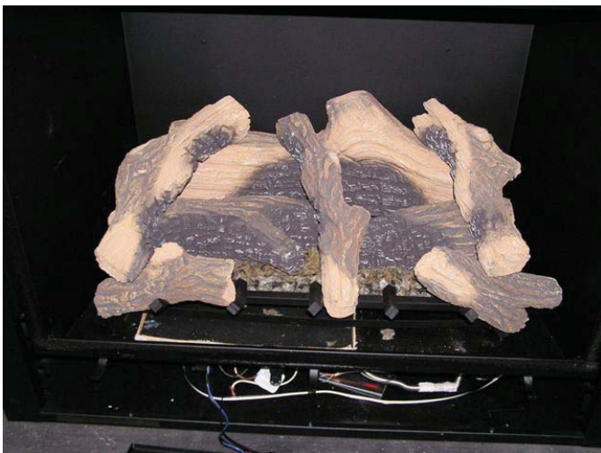
Figure 53 - Installing upper right log
