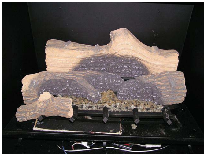
Figure 49 - Installing left front log
